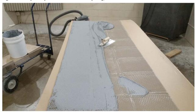
$\overline{\text{Figure } 2 - \text{Pretreatment of tiles with smooth mortar layer}}$
